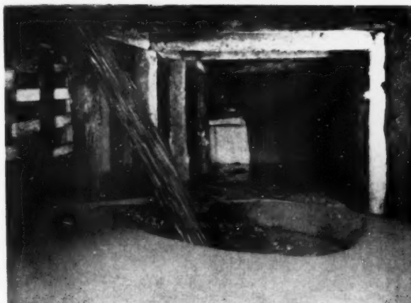
LEFT: Sand filling a mined-out, square set stope at the Frood-Stobie mine of the International Nickel Company of Canada, Limited, Sudbury district, Ontario, Canada. Some 3,000 tons of filling per day is now being placed in stopes down to the 3,100-foot level. RIGHT: Unloading 78-ton railroad cars full of dewatered tailing at the sand-fill mixing plant at the Frood-Stobie mine. The tailing is pulped with water and pumped underground for filling.
